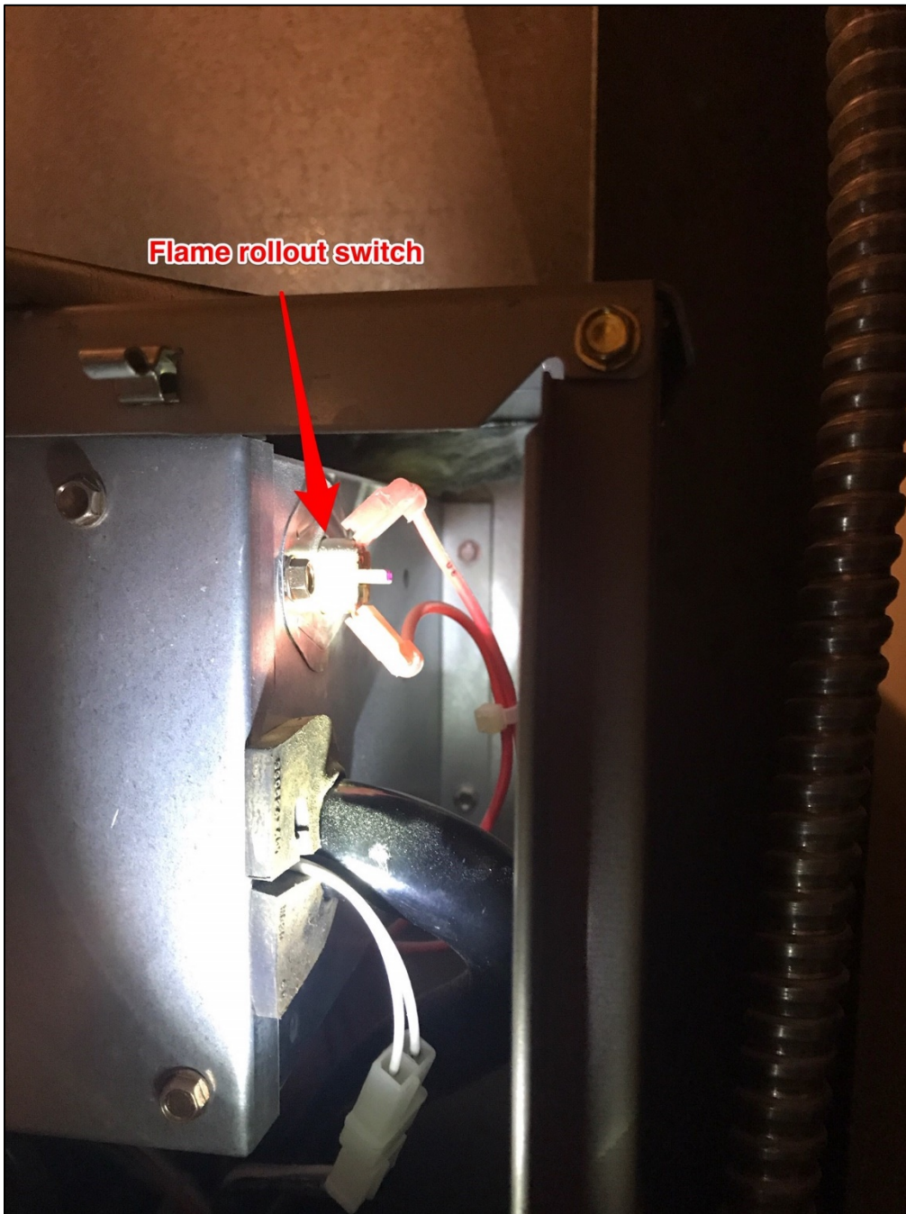
Image 5 - Flame rollout switch on burner box with manual reset button in the middle.
